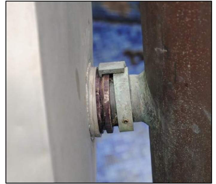
Half round fitting removed shows areas from which 'buckets' leak
