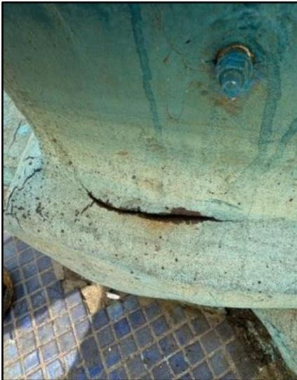
Cracks in existing base
