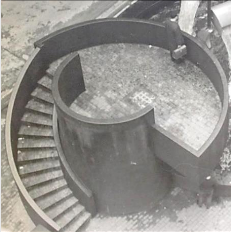
Original brindle red tiling to platforms & stairs Stairs relined with dunbar chequer plate steel
