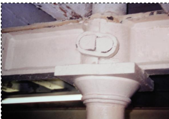
Fig 4 - Method of clamping cast iron beams to the supporting cast iron columns
