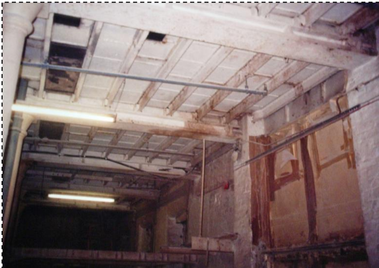
Fig 3 - Underside of iron plate floor on iron joists
