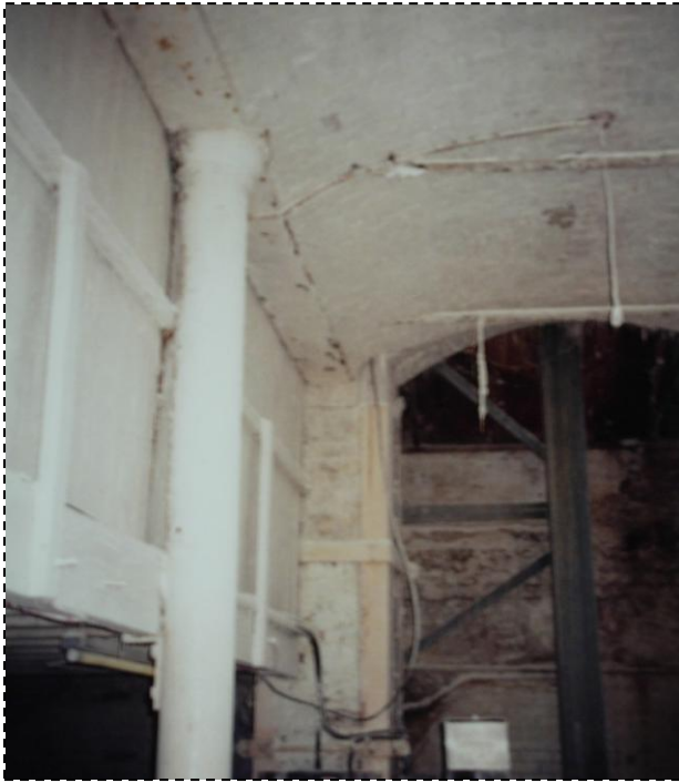
Fig 5 - Cast iron columns with brick arches springing from the cast iron beams and wrought iron ties preventing spread
